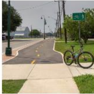
Protected bike lane elevated to curb level
