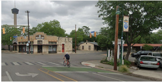
Bike box at the intersection of Alamo Street and Presa Streets positions people biking in front of car traffic which increases cyclist visibility and safety.
