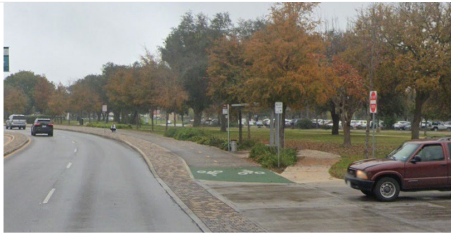
Physically separated bike lanes (or cycle track). Example on Floyd Curl Drive.
