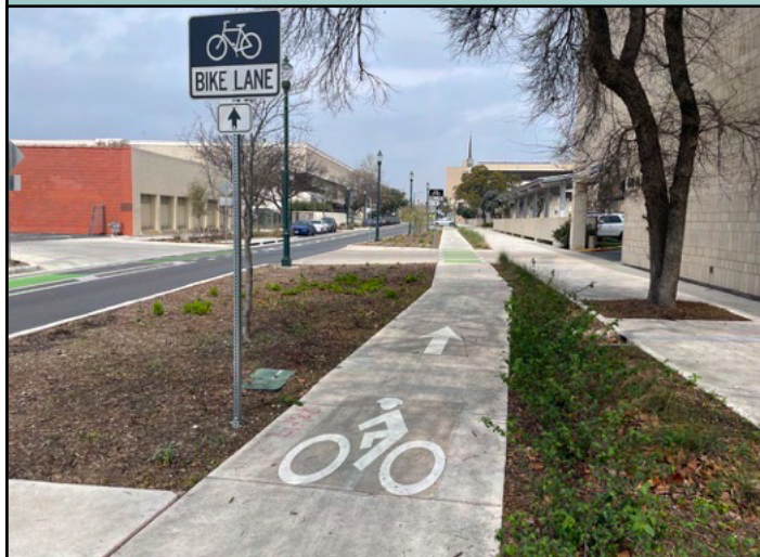
A full-build protected raised bike lane on Main Street in Downtown San Antonio.
