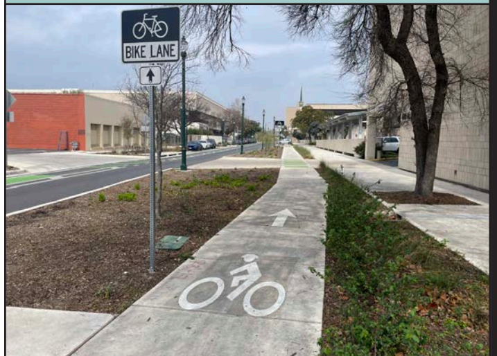
A full-build protected raised bike lane on Main Street in Downtown San Antonio.
