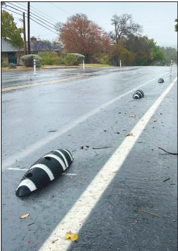
Protected Bike Lanes Installed in Austin, Texas
