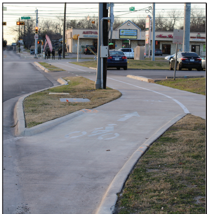
Intersection Bike Lanes Ramps in Austin, Texas
