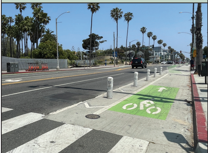
A quick-build type protected bike lane project on Ocean Ave. in Santa Monica, CA.
