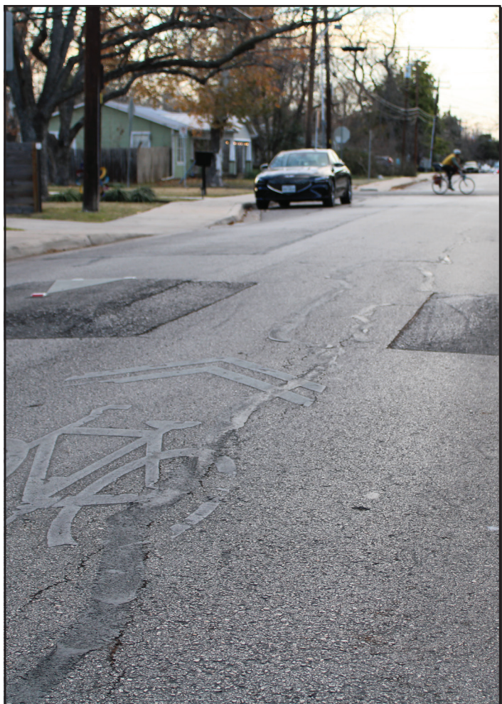
Bike Boulevard on a low-speed street in Austin, Texas
