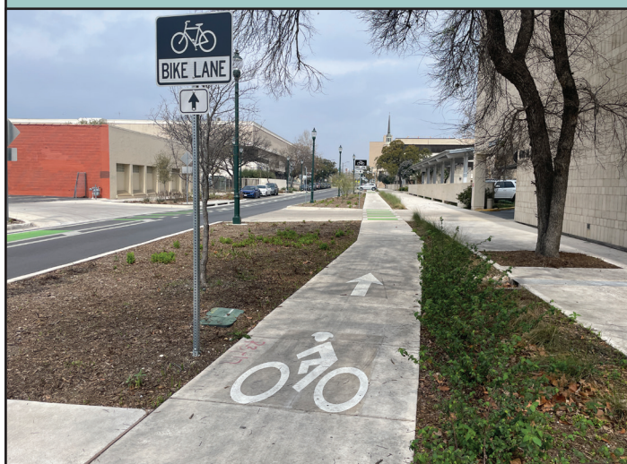
A full-build protected raised bike lane on Main Street in Downtown San Antonio.
