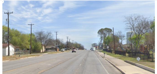
4-foot bike lanes may not provide enough separation from fast-traveling vehicles for people of all ages and abilities to bike along this 35MPH roadway. Example on Gillette Boulevard.
