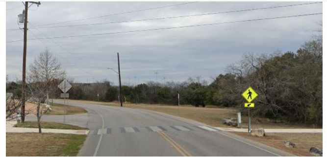
Crossings provide no indication to drivers that people biking may cross. Cyclists can travel significantly faster than people walking and may not be expecting faster cross traffic. Example on Southside Lions Park Trail across Haiwatha Street
