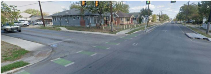
Conflict Markings Through Intersection / Driveway
