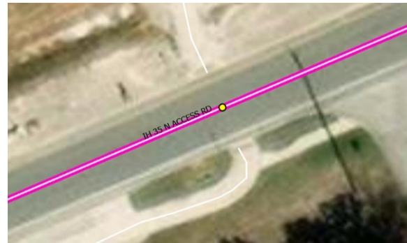
I-35 N ACCESS ROAD AND TRAIL
